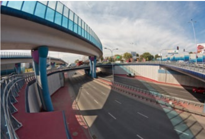
The modernisation of Jerozolimskie Avenue, a section of national road No. 8
