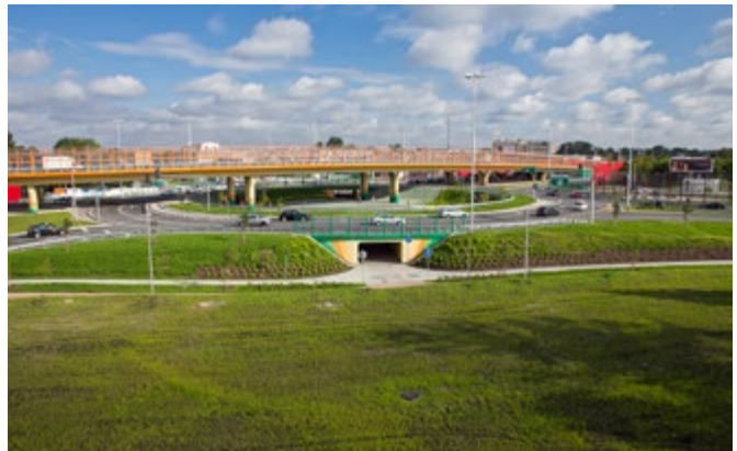
The intersection of national road No. 3 with the Siekierowska Route.
